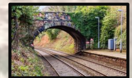
Stone railway bridge
