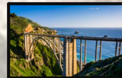
Concrete road bridge
